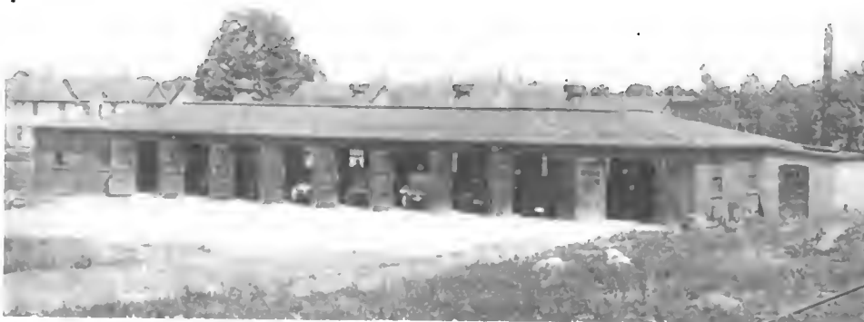
Testing Garage. Where the Cars Undergoing the Road Test Are Sheltered
